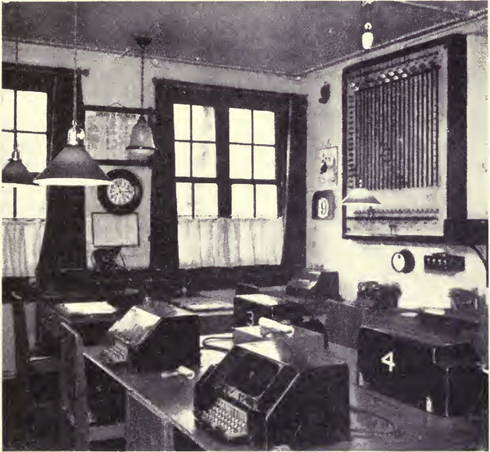
Foreign teletype systems. Central signal room, police headquarters, Amsterdam, Netherlands.
